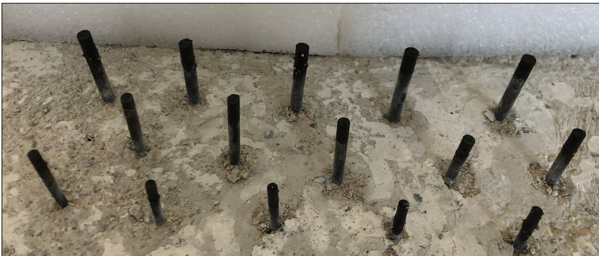
Figure 6- Nails shot at the concrete surface. Back row: 6 mm-diameter nails, middle row: 5 mm-diameter nails, front row: 4 mm-diameter nails.
